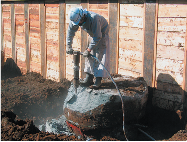
Figure 1 Chipping works by the breaker generating noise and vibration.
