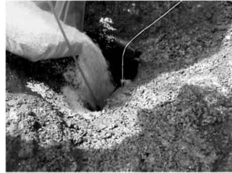
Fig. 3 Loading operation in a wet borehole.
