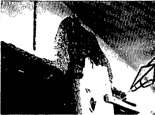
Phot. 1(a) Scabbing of concrete wall caused by gas explosion and the openings of wall from which the whole fittings have been blow away together with windowpanes by the explosion
