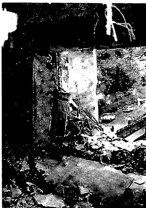
Phot. 3 Another example of gas explosion in building from which all fittings had been blow away together with windowpanes from the opening of reinforced concrete wall
