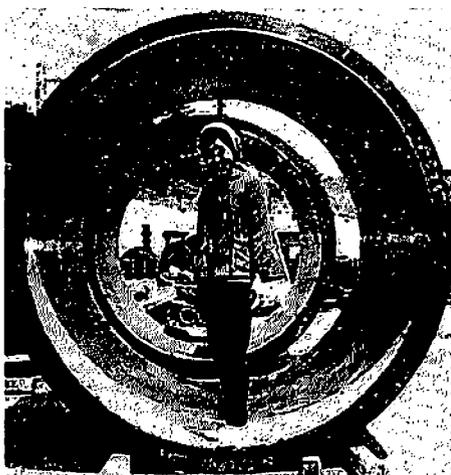
← Photo. 16 Explosive lined cylinder. Liner is titanium 4mm thick. Shell is steel 100mm thick.
