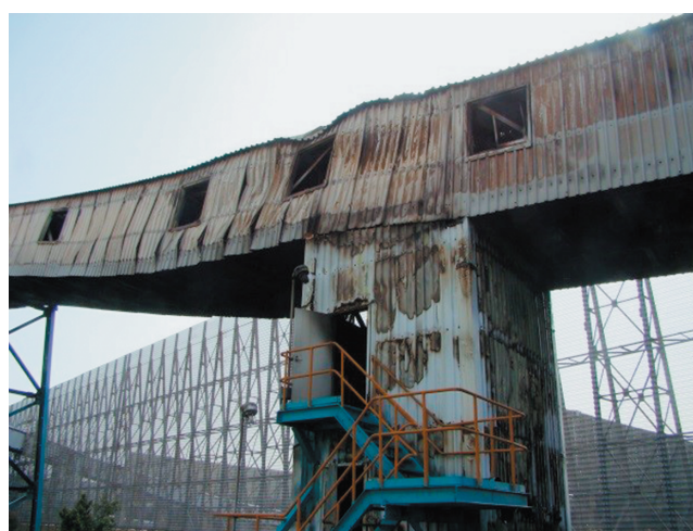
Figure 6 Weighbridge bending from the heat.
