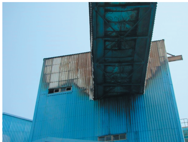
Figure 5 Tower TR9 showing discoloration.
