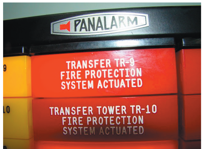
Figure 20 Fire alarm control panel located in the control center.
