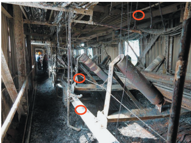
Figure 18 Layout of the sprinkler in Taichung power plant.
