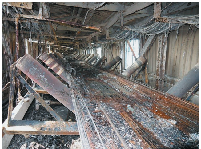
Figure 12 Conveyor belt remains.
