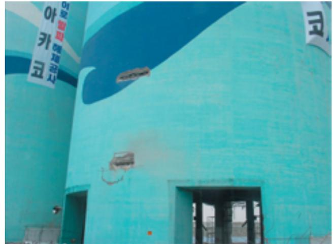
Fig. 6 Slots for leading tension failure and bending failure.
