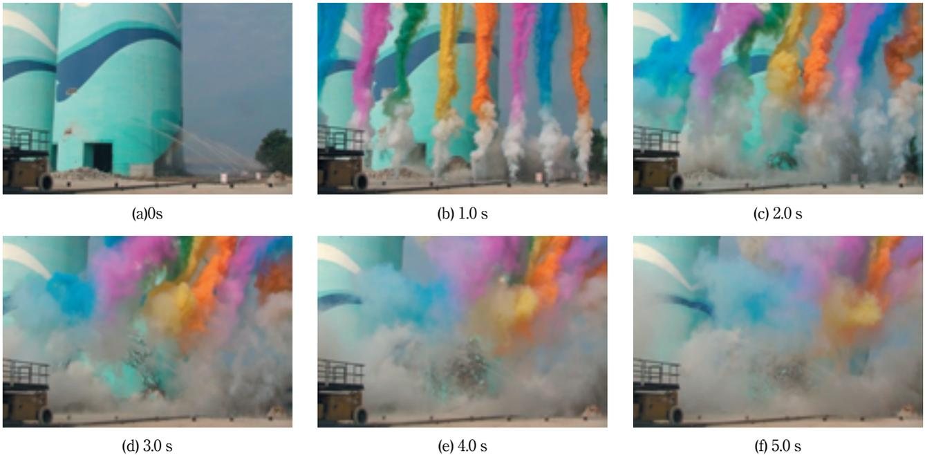
Fig.13 Time–sequence pictures of the collapsing movement of silo.
