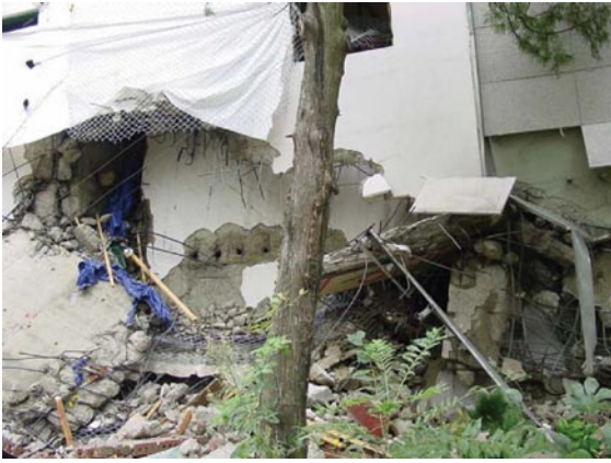
Fig. 14 Picture after blasting of the elevator room.
