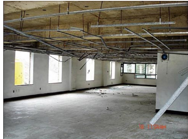
Fig. 2 Inside of the building.
