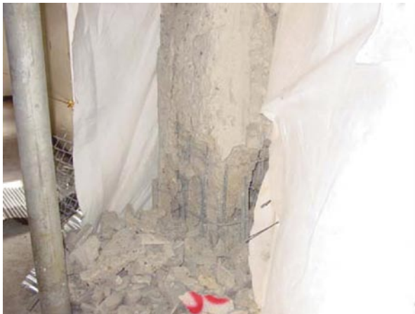
Fig. 8 Results of demolition after the test blasting of the pillar part.
