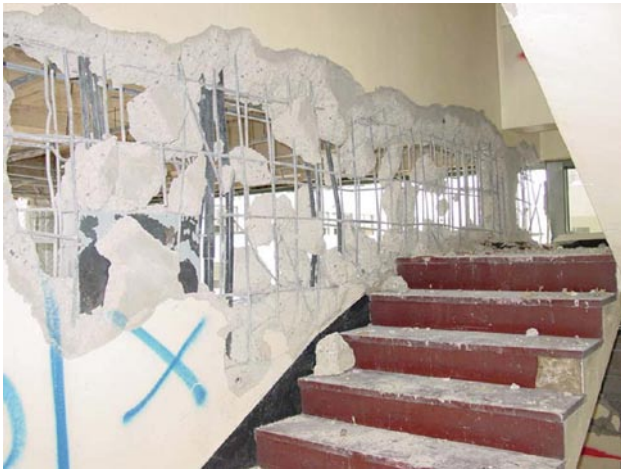
Fig. 4 Picture of the stairs room after weakening process.
